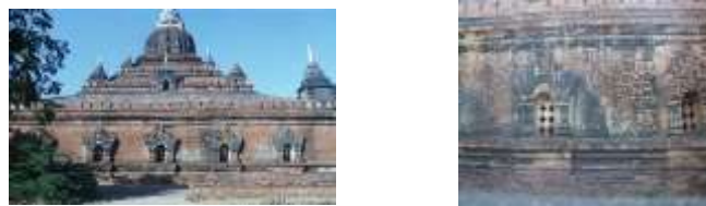
Figure 2. Five Perforated Windows at Nagayon Temple
